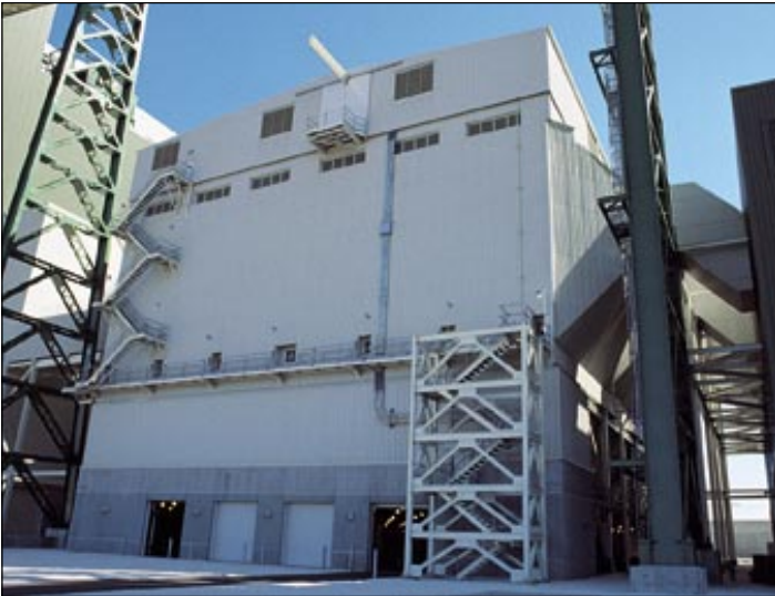
435-megawatt coal-fired power boiler
