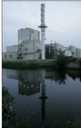
Wood-waste-fired cogeneration facility
