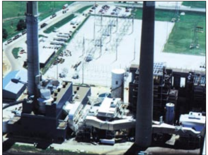
Precipitator and Wet FGD System controls emissions from two coal-fired boilers producing 440 megawatts of power
